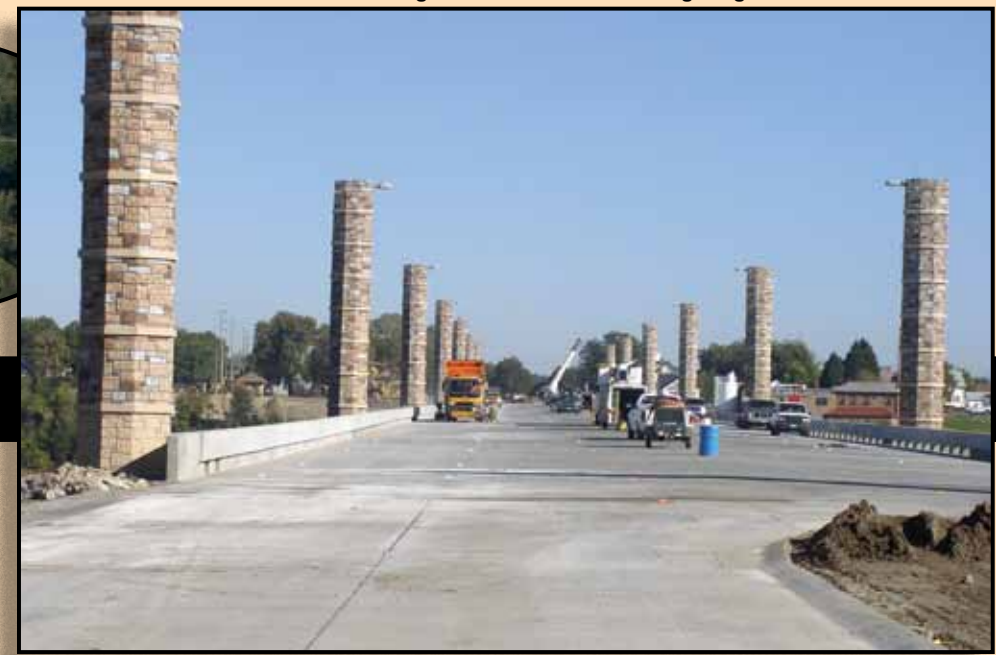
Installation of final cap piece.
